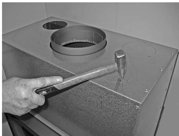
Energa 70-55 Tunnel (Openingen diagonaal open maken.)
